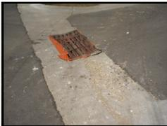
Inlet Protection used to keep sediment out of storm sewers
