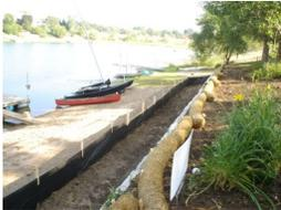
Silt fence and straw waddles can be used to contain sediment on resident's property to keep sediment out of the lake.
