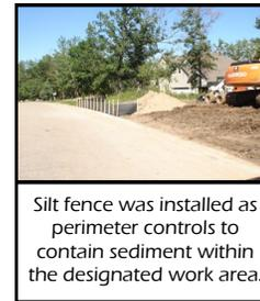
Silt fence was installed as perimeter controls to contain sediment within the designated work area.
